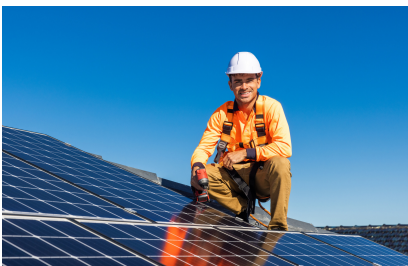
Solar Panel Installation
